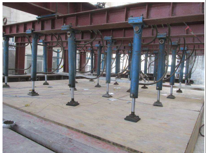
Photo 14: The unexposed surface of the specimen after test duration of 15 minutes
