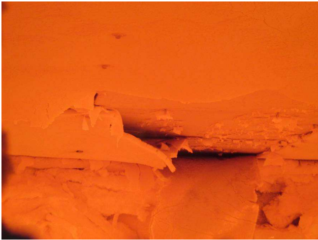
Photo 21: The exposed surface of the specimen after test duration of 62 minutes, showing part of first layer plasterboard ceiling was falling into the furnace
