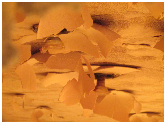
Photo 16: The exposed surface of the specimen after test duration of 19 minutes, showing the lamp cup of specimens fell out from the light can
