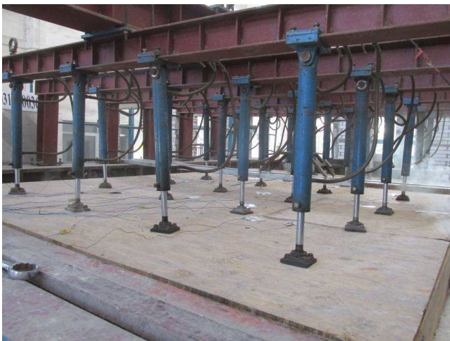
Photo 23: The unexposed surface of the specimen after test duration of 75 minutes.
