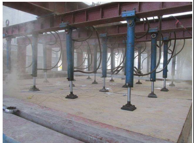
Photo 24: The unexposed surface of the specimen after test duration of 90 minutes
