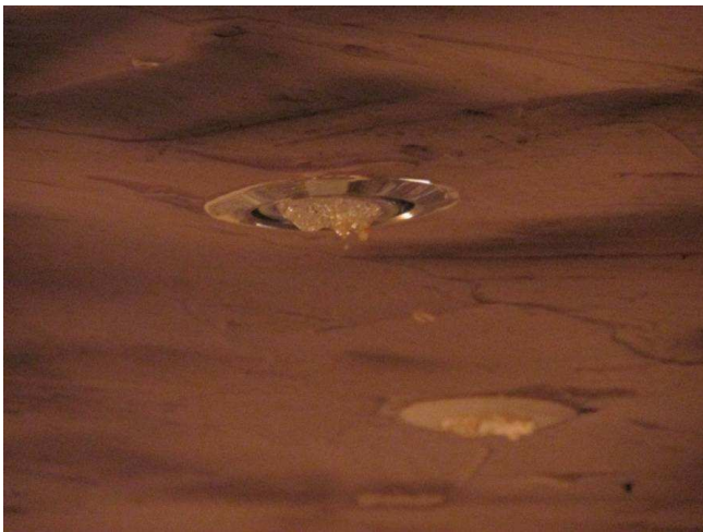
Photo 13: The exposed surface of the specimen after test duration of 3 minutes, showing the lens of specimen was fusing.
